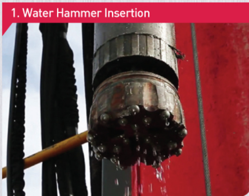
Rig operation/water hammer connected & water pump running
